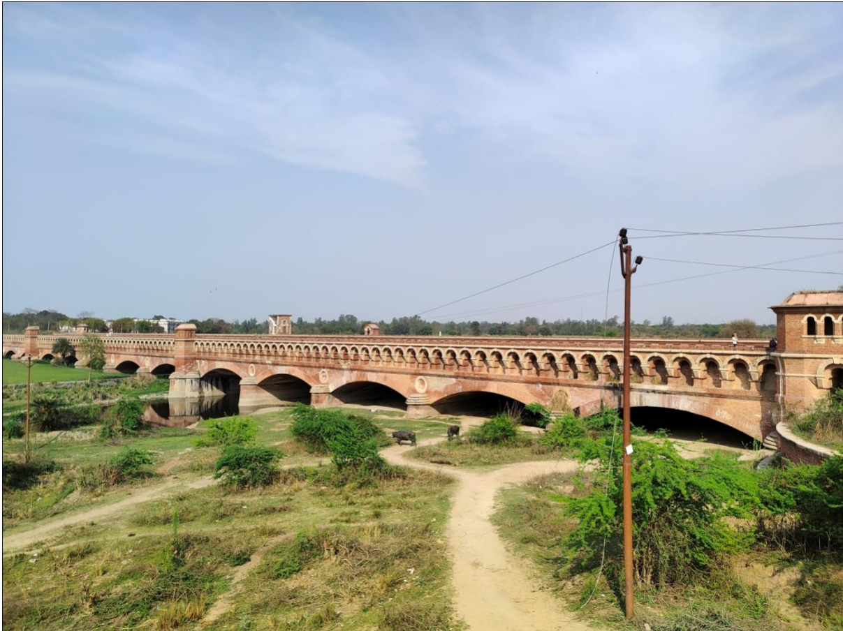
Figure 49. Nadrai Bridge, Image Source: INTACH Team
